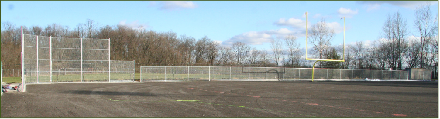
Pleasant Valley Fields ready for turf installation.
