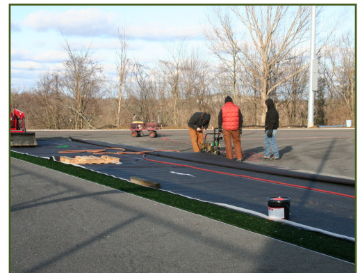
Turf installation begins
